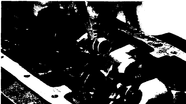
O-Ring at Pump Inlet
